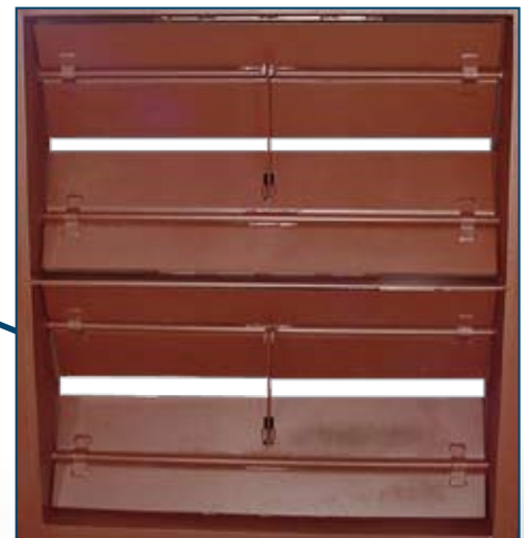
Opposed Damper Blade Design
