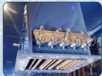
View of Flow Control Vanes
