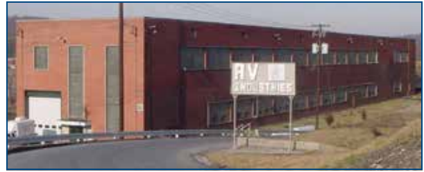
Morgantown Manufacturing Facility
