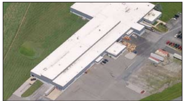
Honey Brook Manufacturing and Warehouse Facility
